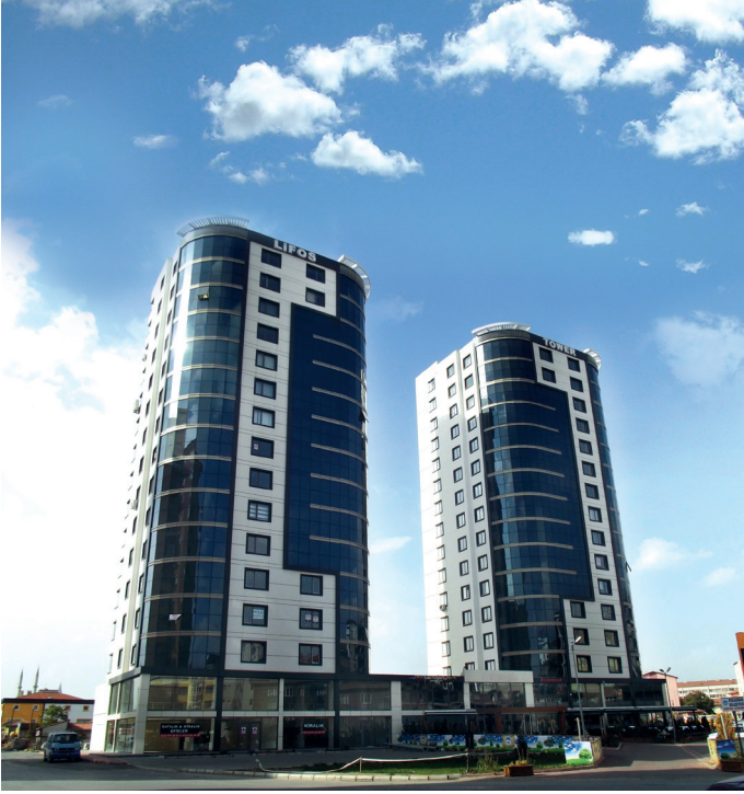
LİFOS TOWER KAYSERİ
